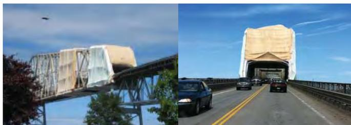
SR 433 – Lewis and Clark Bridge, in Longview. These pictures show the containment for the painting operations on the main steel truss spans. Construction began in 2010 and is scheduled to be complete in 2013.
